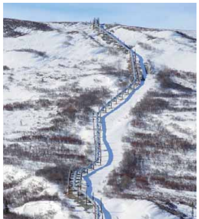
The Trans-Alaskan Pipeline.
